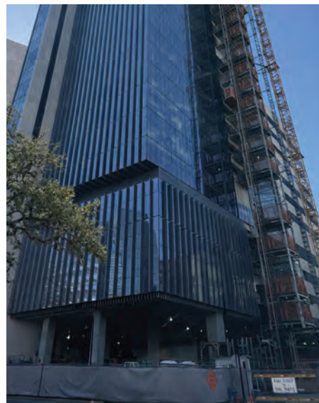
Fig. 1. A column-free northwest corner was needed to accommodate the drive and ambulance parking, and to avoid the underground utilities.
