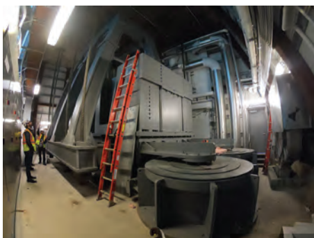
GERB Double Pendulum Tuned Mass Damper
