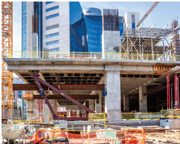
Fig. 7. Temporary supports were required during construction. (Photo courtesy of Vaughn Construction.)
