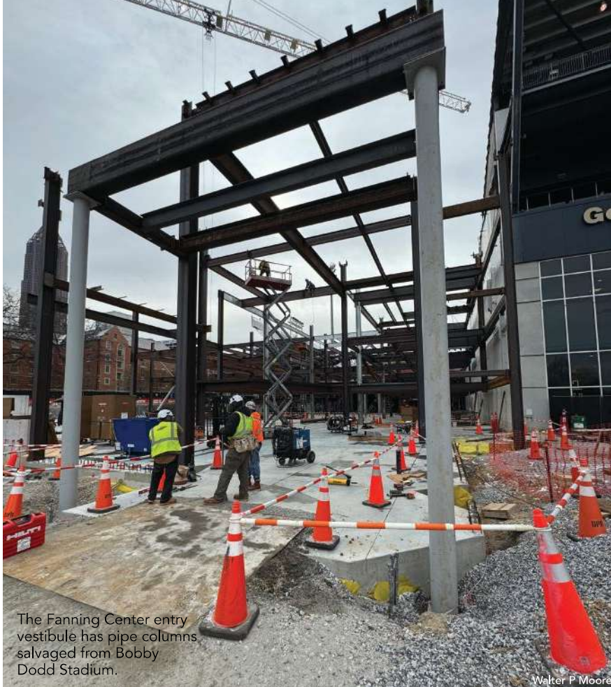
A reused and refabricated column in place in the Fanning Center framing.
