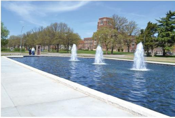
Fig. 6: Delbert J. Haff Circle Fountain after renovation
