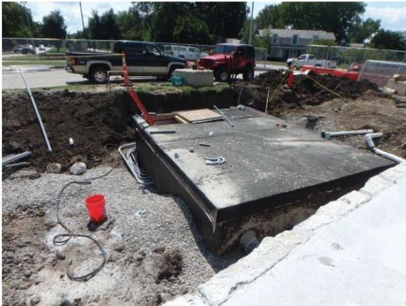
Fig. 10: Installing new underground concrete vault
