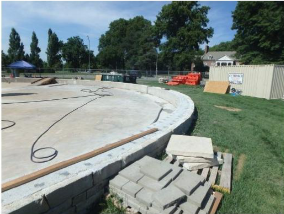
Fig. 9: Creating slope at top of perimeter wall using concrete overlay
