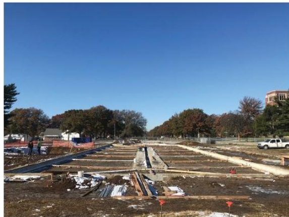
Fig. 5: Construction of new slab-on-grade
