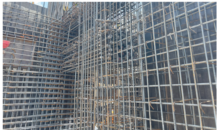
Rebar placement at the outrigger sections as seen in the field.
